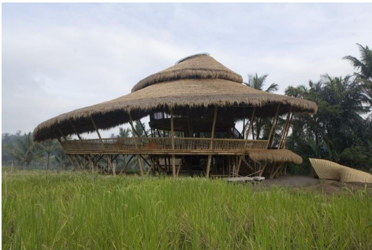
Fig 1.4: Thatched Roof Bamboo
