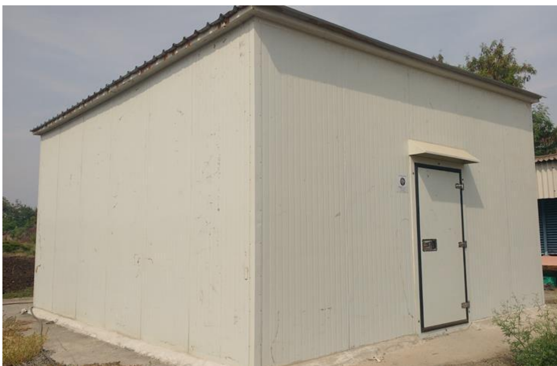
Fig 1.6: Controlled onion storage structure
