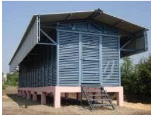
Fig 1.5: Bottom and side ventilated storage structure
